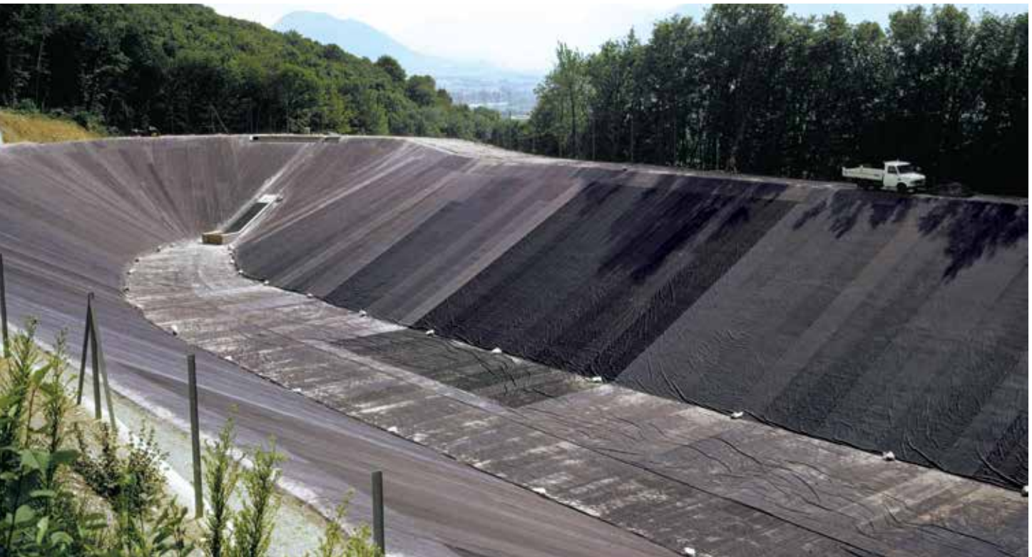
FIGURE 11 Completed installation of the butyl rubber geomembrane primary liner.
