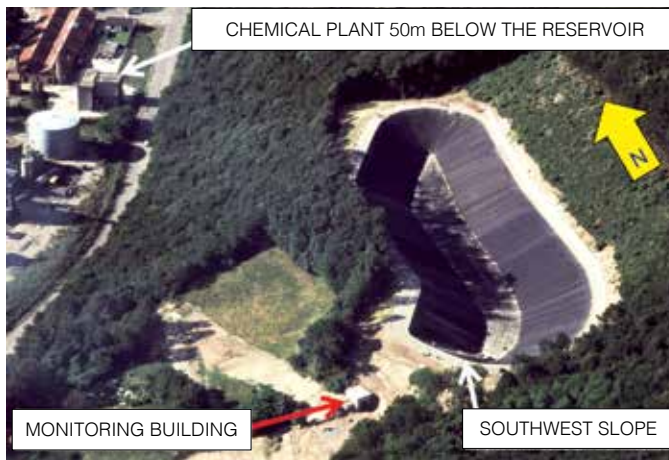
FIGURE 2 Aerial view at the end of geomembrane installation. The shape of the reservoir minimizes the impact of excavation on the stability of the east slope and the weight of the dike on the west slope. The reservoir proportions are distorted because the photo was taken at an angle (as evidenced by the fact that the intake structure on the 1V:2H southwest slope is hardly visible).
