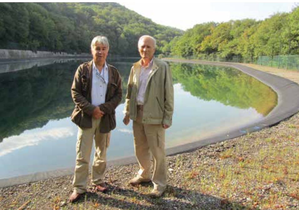
This photo, chosen by the Geosynthetics editor, shows JPG x 2 (J.P. Giroud—right, J.P. Gourc—left) at the first double geomembrane lined reservoir, designed and constructed in 1973–74 near Grenoble, France.
