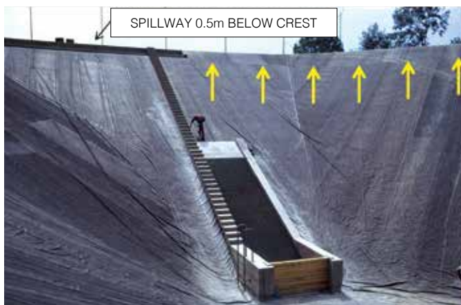
FIGURE 3 Southwest end of the reservoir showing: water intake structure, spillway, and butyl rubber geomembrane. The butyl rubber geomembrane is unreinforced, except at the top of the slope where a strip of reinforced butyl rubber geomembrane is used around the entire perimeter (except at the spillway) above the level marked by the yellow arrows and in the anchor trench.
