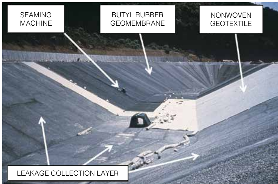
FIGURE 10 Installation of the butyl rubber geomembrane primary liner on a geotextile.
